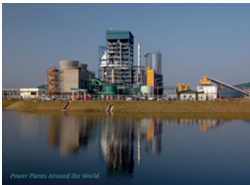
Figure 7 Rice husk based power plant in Thailand
